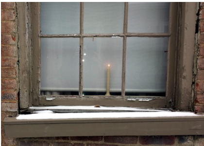
Examples of window conditions on the west side of Highland House before replacement.
