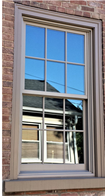
West side replacement window. (Window sill constructed of concrete for a longer lasting solution.)
