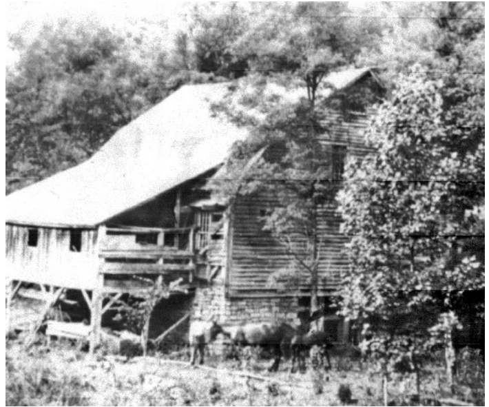
A view of the east side of the Porter Mill circa 1920s. The mill was permanently closed in 1914 after new technology made stone ground grist mills obsolete. It is believed the person in the picture with the horses is Walter "Buddy" Porter, the last owner. Behind him you see the cut stone foundation and stone walls for the mill. The water wheel was located at the right north-east corner of the mill. The area where the horse is standing would have been the pool and tail water, after the water passed over the water wheel.
