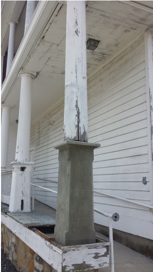
(left) New concrete pillar in back of house. (right) New patio for A/C units. (below-left and right) Underground tile will carry rainwater away from the house.
