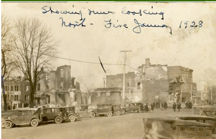
Aftermath of the 1928 Murphy-Benham fire. North High Street is to the right.
