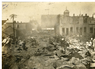
(below) Back view of the 1908 Barrett Livery Fire
