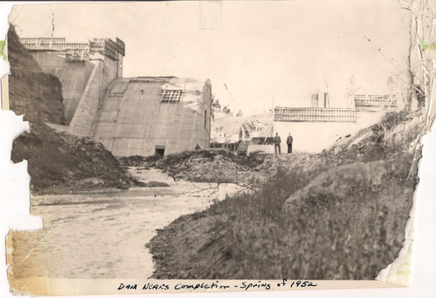
Rocky Forms Dam near completion, Spring 1952
